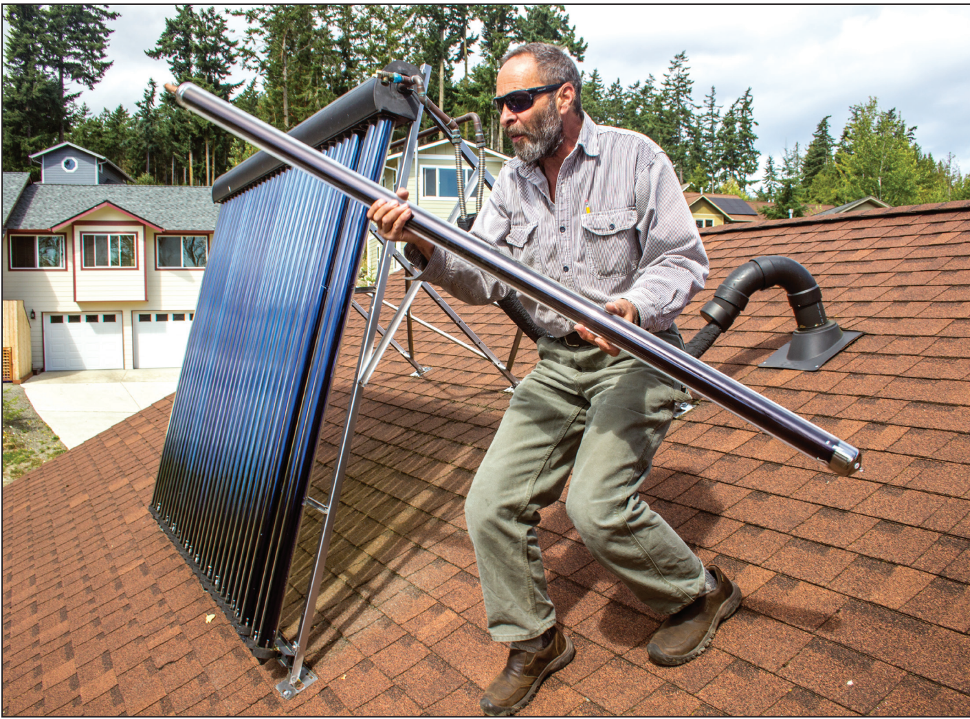
Kenny Schordine, owner of Solar Hot Water of Port Townsend, makes repairs to a passive solar hot water heating system he installed about eight years ago on top of a Port Townsend home. Each solar tube is surrounded on the outside by a transparent layer of glass. The next layer is a nearly opaque layer of glass. The center is hollow and includes a copper heat pipe through which coolant flows. Heat from the tubing is transferred through piping into a water heater in the garage. Leader photos by Chris McDaniel
